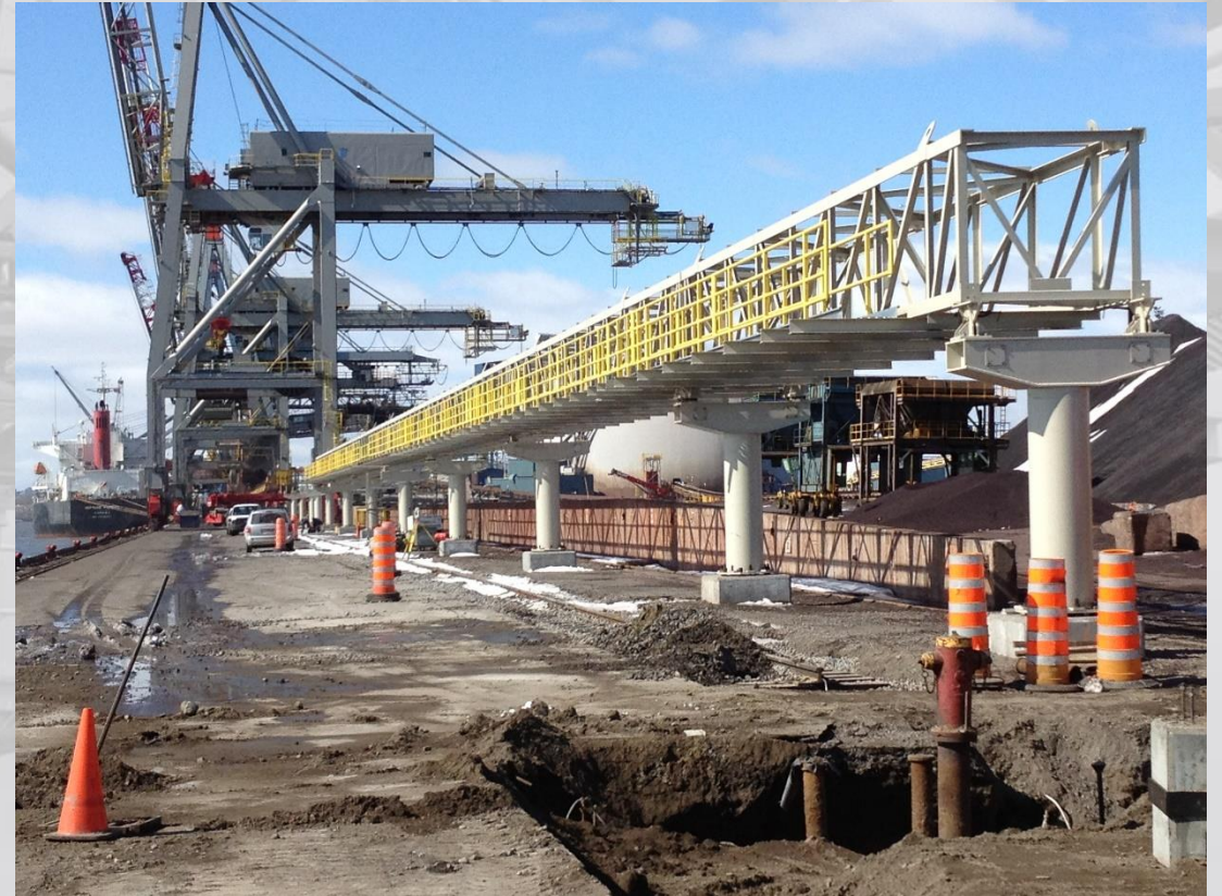
Transfer conveyor, Beauport QC (60" wide, 3500 TPH, 75' span)
